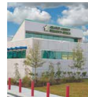
Orange County Sheriff's Office Building Sector II
